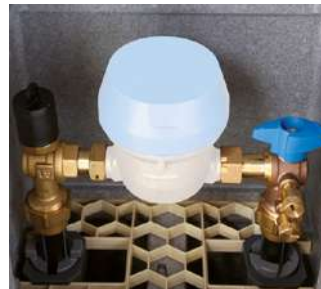
45K Before water meter valve tamper-proof + valve-check valve (elbow)
