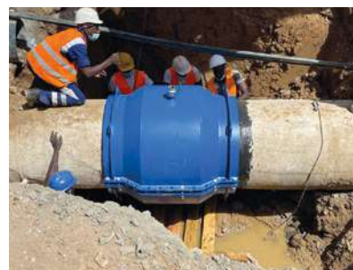
Repair of large-dimension pipes in buried networks or in pumping stations.
