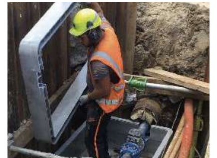
Modular chamber installation
