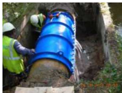
Repair of large-dimension pipes in buried networks or in pumping stations.
