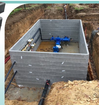
Modular chambers for faster and safer work
