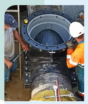
Installation of a 3D ND 600 valve on welded steel helical pipe. Under-pressure drilling without any disruption. The canal can now by isolated from the lake and the risk of polluting the river has been eliminated.
