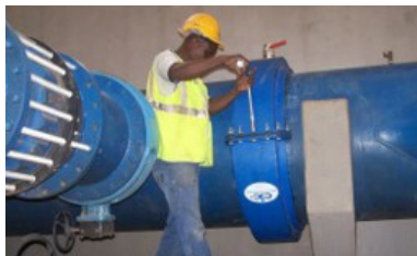
Repair of large-dimension pipes in buried networks or in pumping stations
