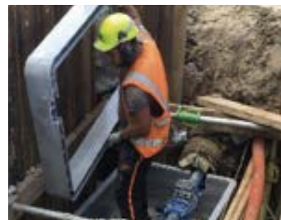
Modular chamber installation
