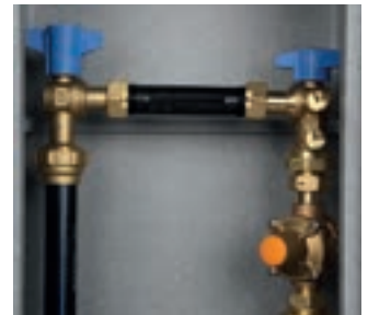
Assembly with pressure reducer
